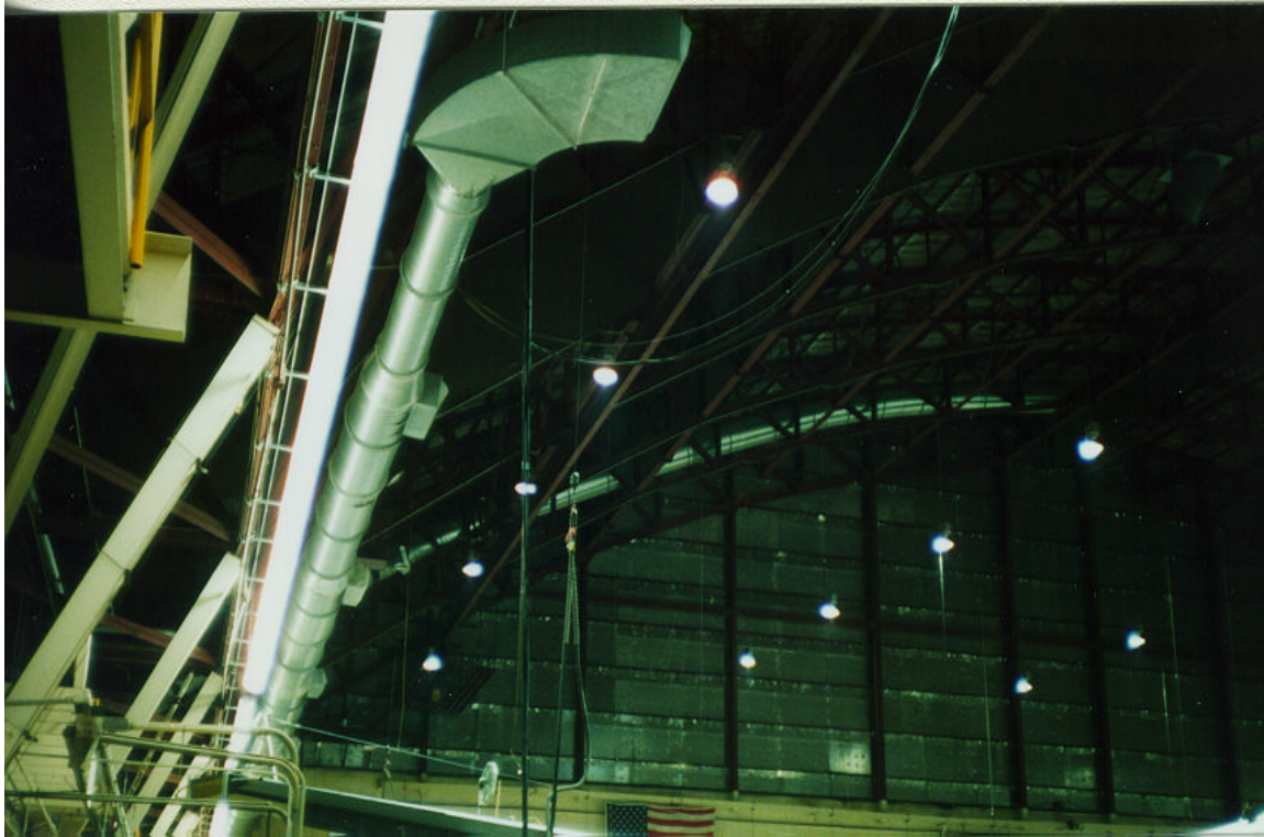
Figure 12. Pre- (top) and Post- (bottom) Retrofit in High-Bay - Added Edge Light Pipe
